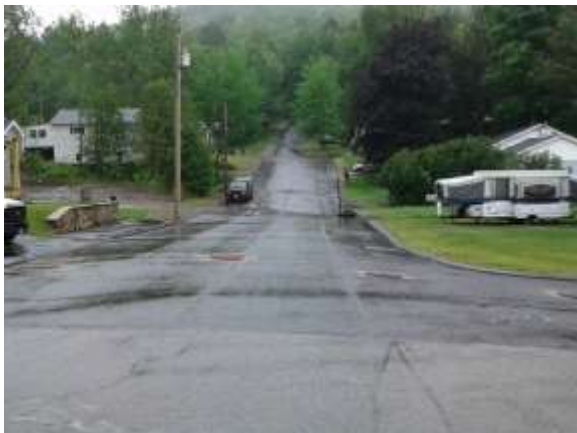
*Howland Street Repaired
