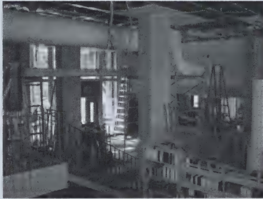
Installation of the new ductwork and ceiling
