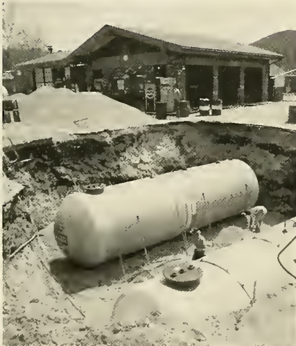
Gas Tank Inspection.
