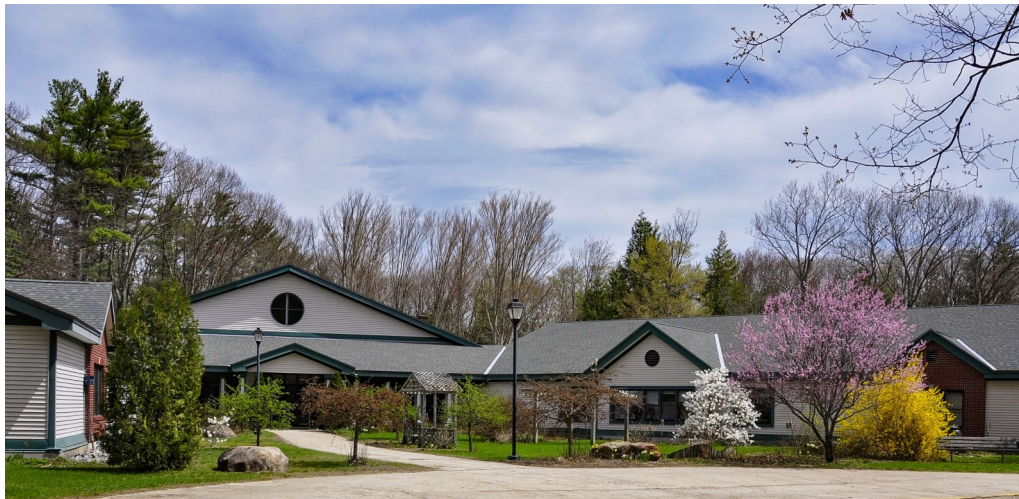
Francestown Elementary School
