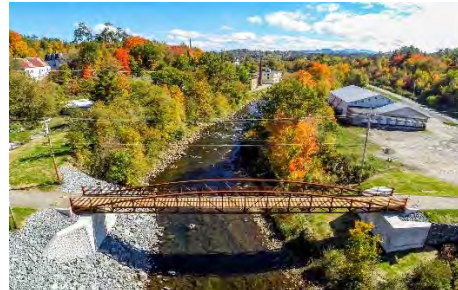
Multi-Modal Bridge (Bridge Street)
