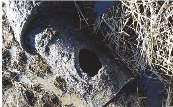
The discharge of this untreated waste resulted in the closing of the clam beds in the harbor. By mid-march we had hired a contractor, built a temporary road 1,500 feet out into the marsh, and replaced a 10-foot-long section of the pipe. The cost of the repair was approximately \$135,000.
