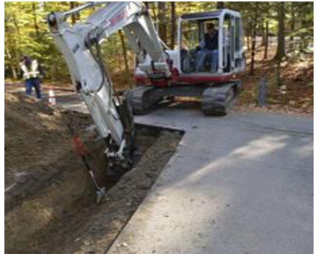
Repair of Culvert at 33 Sanborn Road
