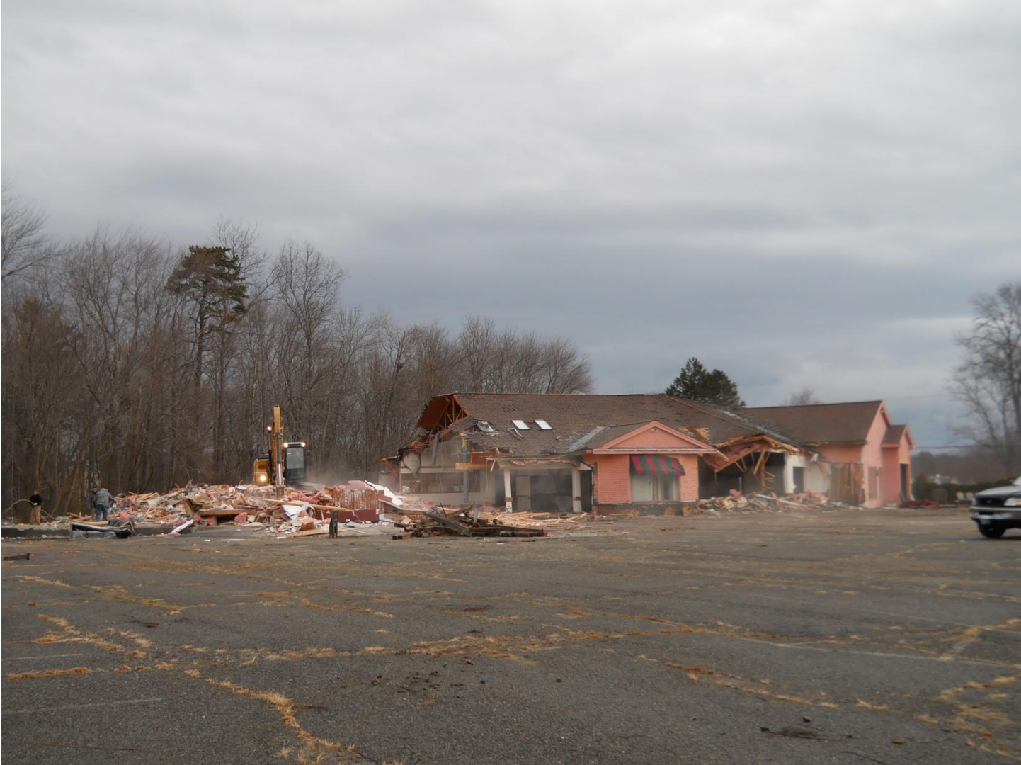
Demolition of the former Faro Gardens function establishment at 11 Lafayette Road.
