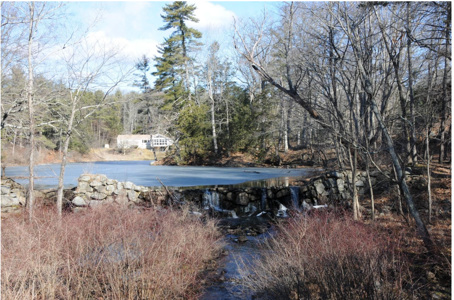
View from the Old Stage Road Bridge
