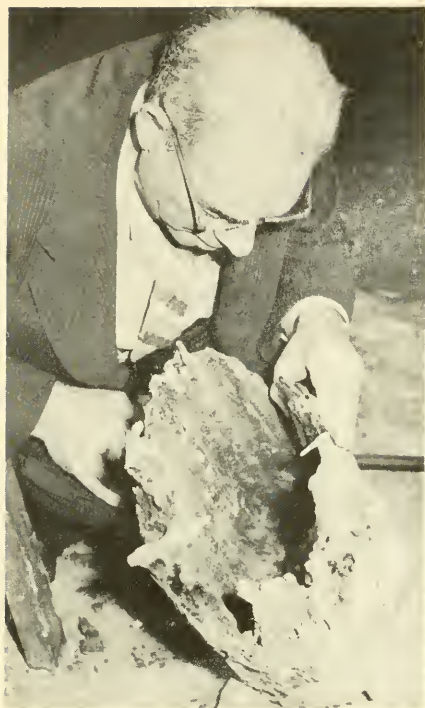
(Left) Old wooden pipe dug up during the reconstruction of Main Street. (Below) Timber cut at Long Pond is stacked and stored for later use.
