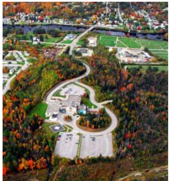
Northern NH Correctional Facility (Eric Kaminsky)
