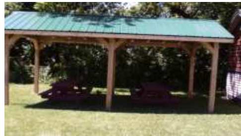
Community/Central Park Shelter
