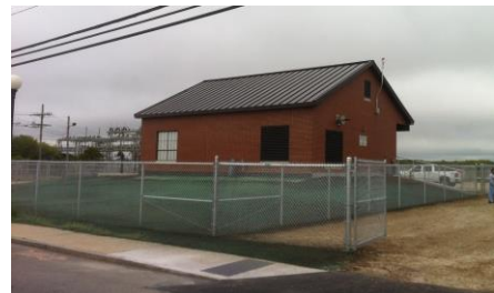
Church Street Pump Station
