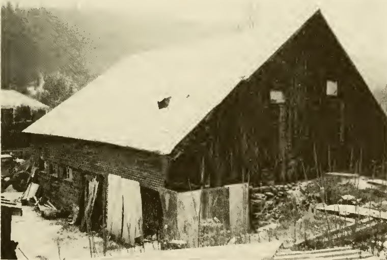
EXISTING HIGHWAY GARAGE FACILITY - Photo by Dick Gassett
