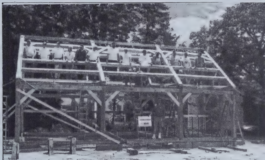
Framing the Bradford Blacksmith Shop
