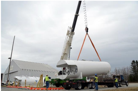
Jet-A Fuel storage tank being put in place
