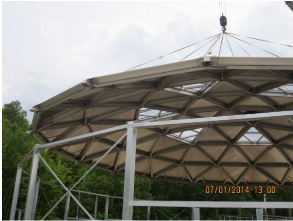
Secondary1 Dome Cover coming into place
