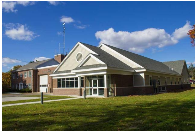
(Newly constructed Winnacunnet Rd)
