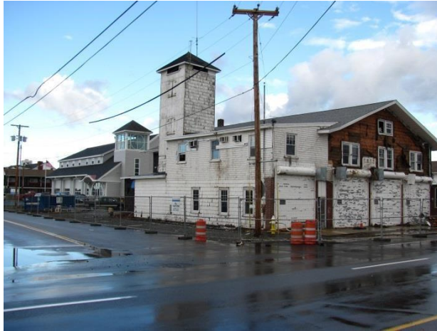
(Ashworth Ave Station on demolition day)
