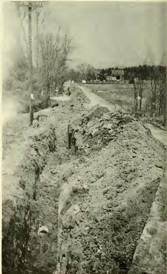
Preparations for Installation of Water Line on the Durham Road and Bellamy Road.
