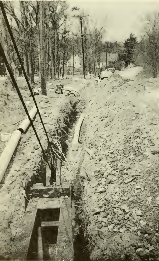
Preparations for Installation of Water Line on the Durham Road and Bellamy Road.
