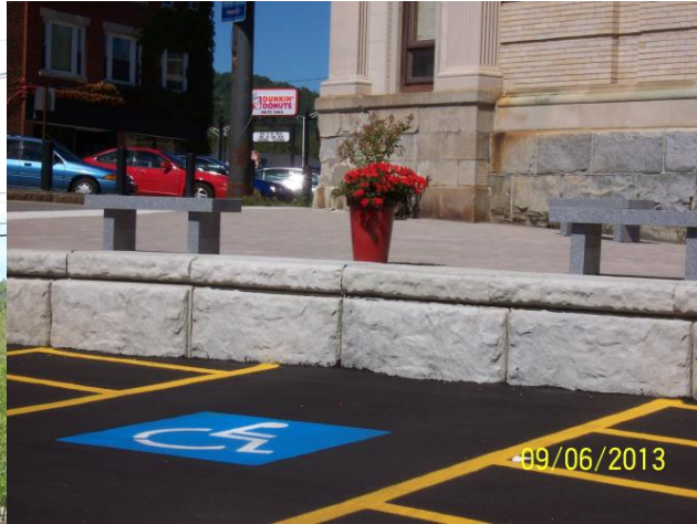
3 Glen Avenue... after
