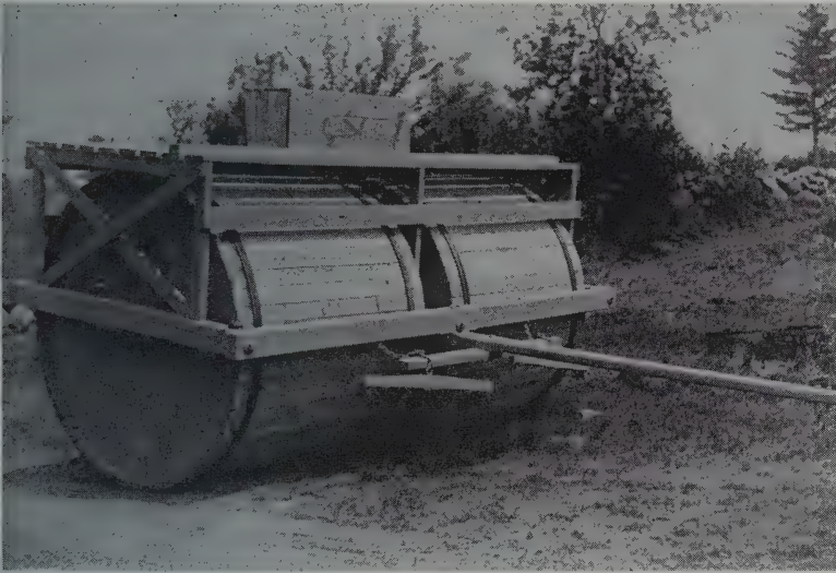
Sutton's Snow Roller, built by J. H. Keyser
