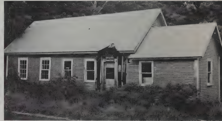
CHANDLER BROOK SCHOOL Owners: State of New Hampshire
