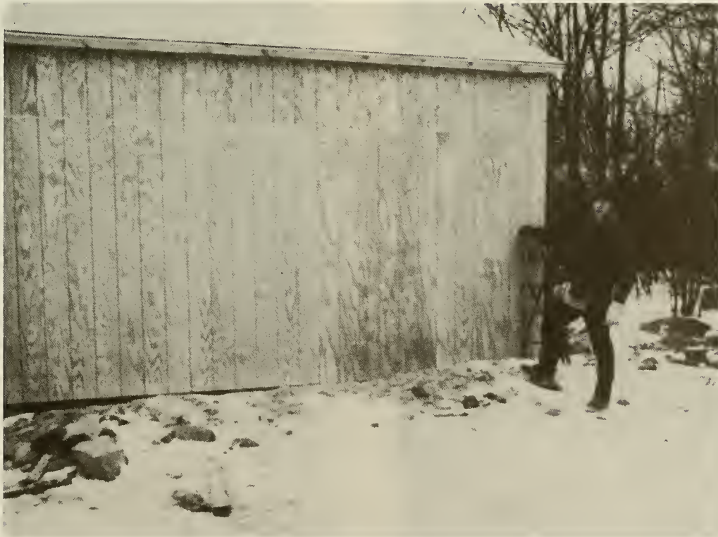
NEW BUILDING TO HOUSE 1930 SEAGRAVES TRUCK
