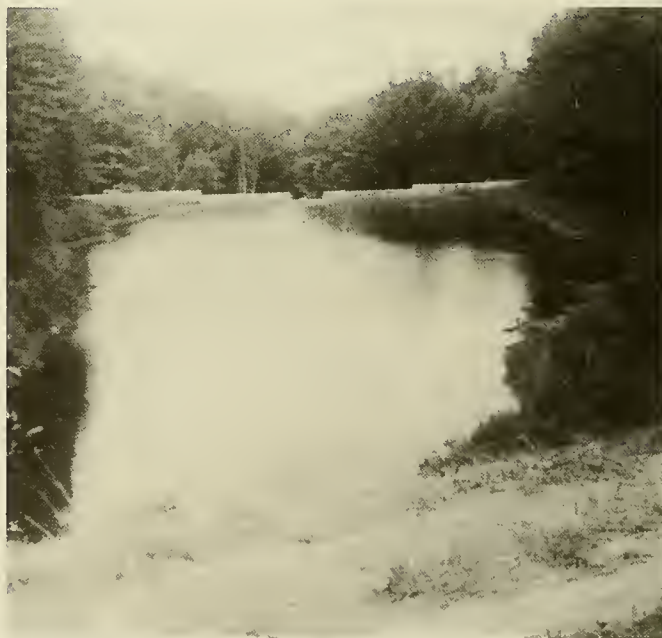
Goffstown's Lower Reservoir located on Uncanoonuc Mt. Capacity 9,000,000 gallons
