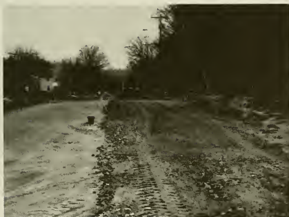
Folsom Road Reconstruction
