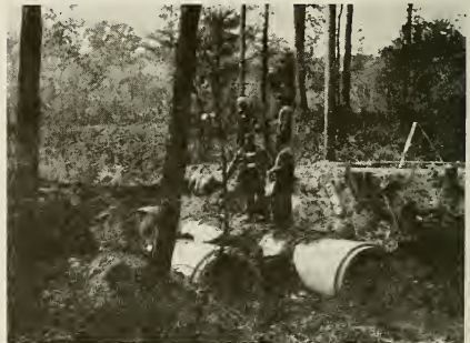
Mill Road Construction
