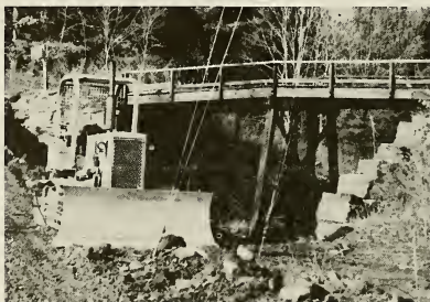
Madden Road Bridge
