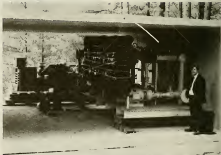
Scobie Pond Road Water Pump Station
