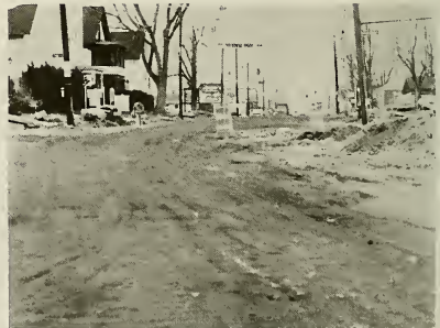
East Broadway Reconstruction
