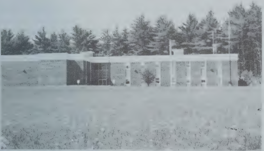
Carroll County Administration Building • Route 171, Ossipee, NH
