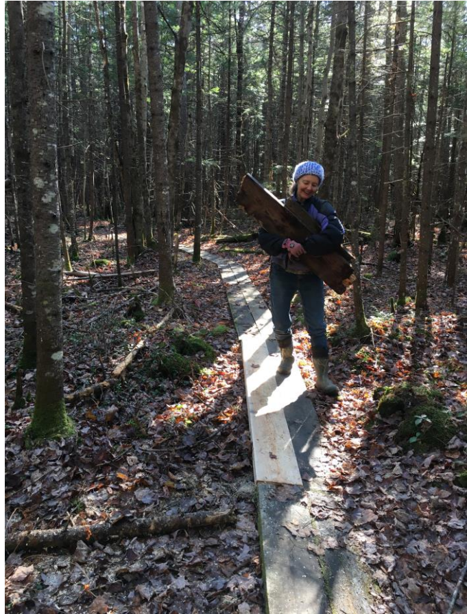
Annual Bradford Boardwalk Repair Day Photo by J. Ann Eldridge
