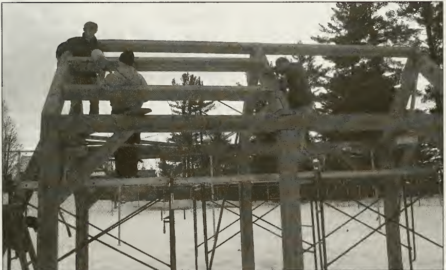
Building of Pavilion
