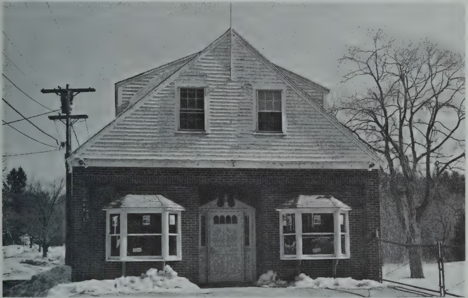
Plaistow's new Historical Museum, formerly the Plaistow Fire Station, Main St.
