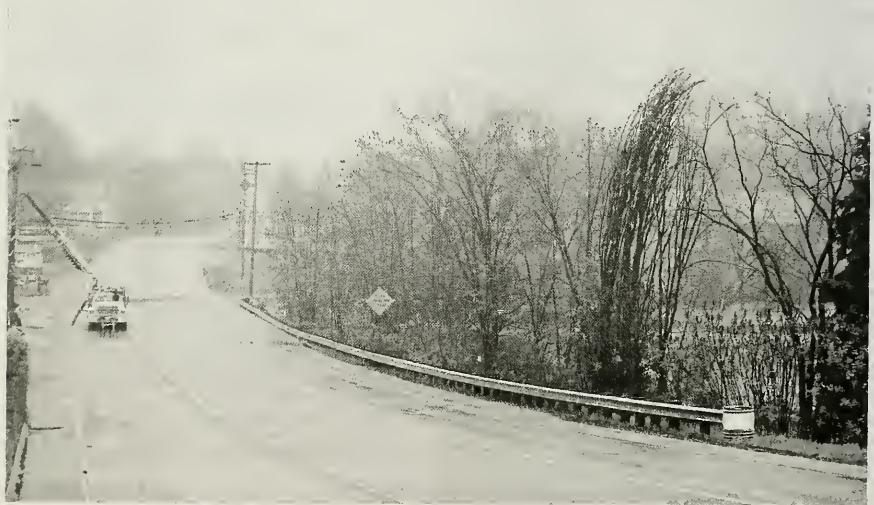
Flooding over Route 1 from Whittier Pond May 11-13, 2006
