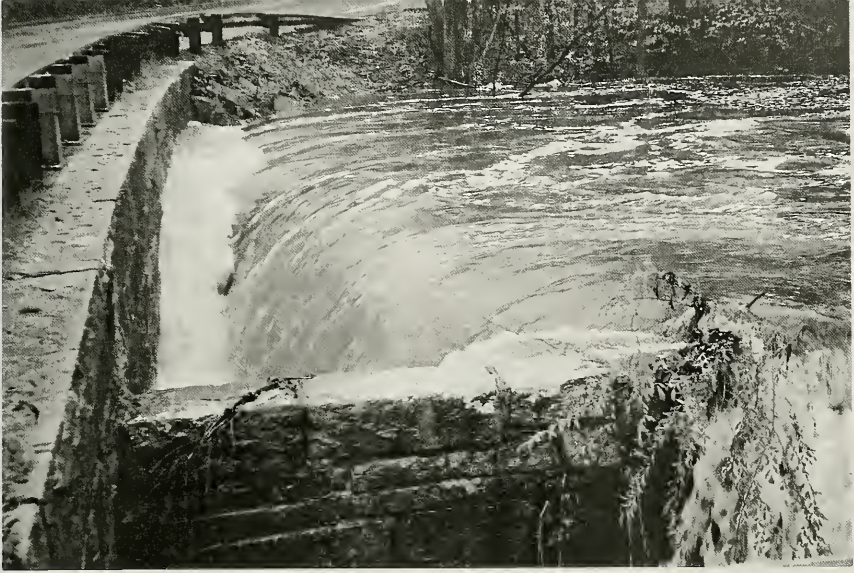
The May floods demonstrate the power of nature as the water surges under Route 84 at the Falls May 12, 2006
