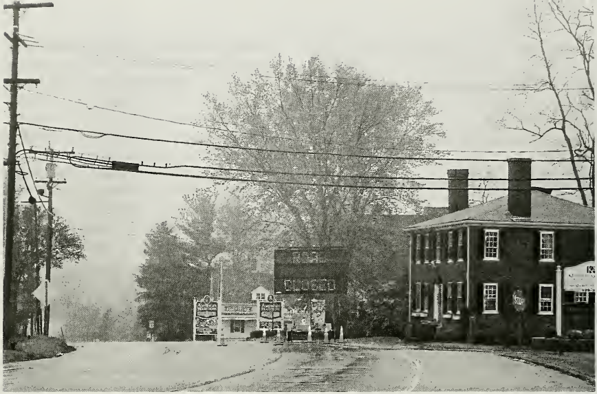
ROAD CLOSED sign near Route 84 and Route 1, May 11-13, 2006 No traffic was allowed for several days due to the floods below at Whittier Pond
