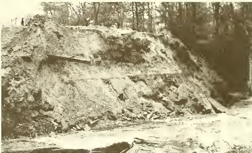
Railroad Retaining Wall
