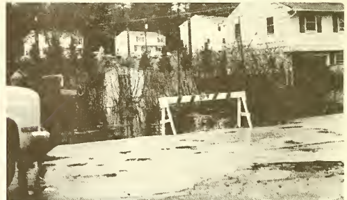
Bradford Street Bridge
