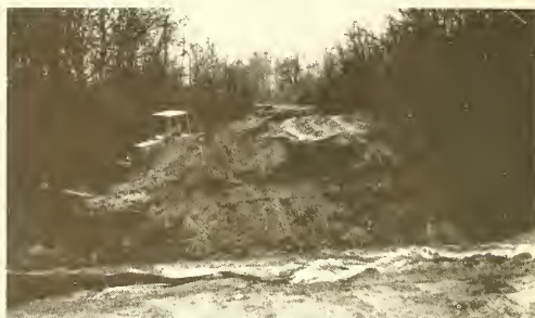
Railroad Retaining Wall
