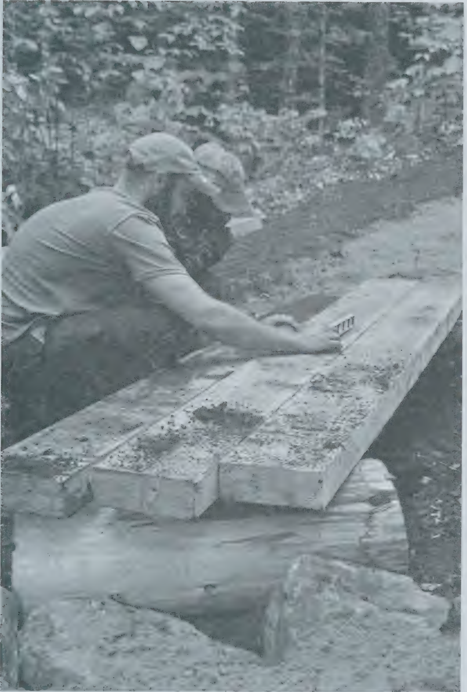
Checking the grade creating a bog bridge to Rollo Falls
