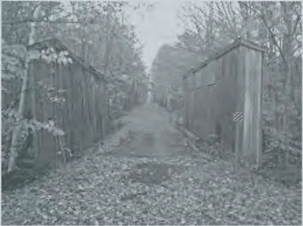
Howe Pony Truss Bridge
