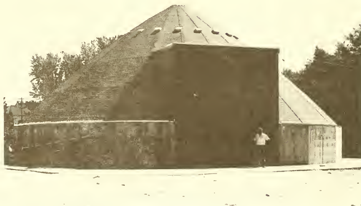
New Salt Storage Shed
