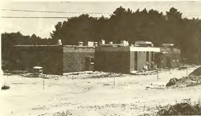
Wastewater Treatment Control Facility
