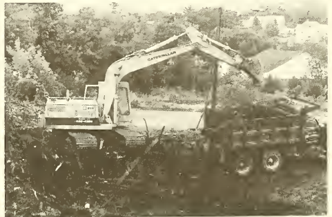
Demolishing burned out building on Merchant's Row
