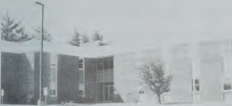
The Carroll County Administration Building, which has the Sheriff's Department, Registry of Deeds, Probate and District Courts, and offices for the Commissioners, Treasurer and Business Office.
