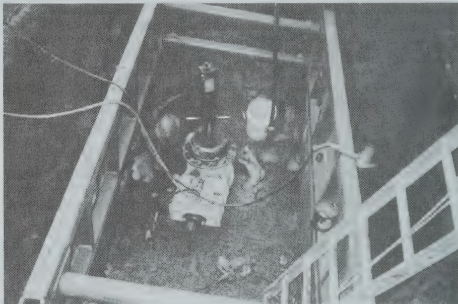
Water Main Valve Installation on Plymouth Street
