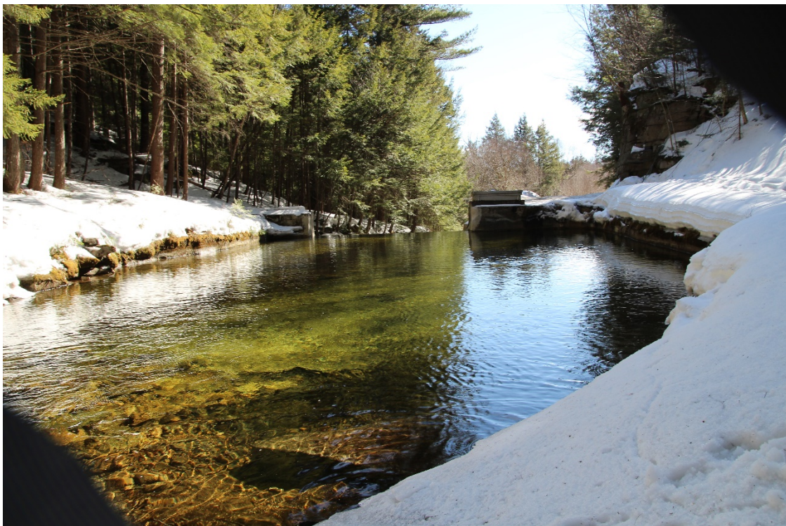
Perkins Brook Dam Photo courtesy Normand Jacques
