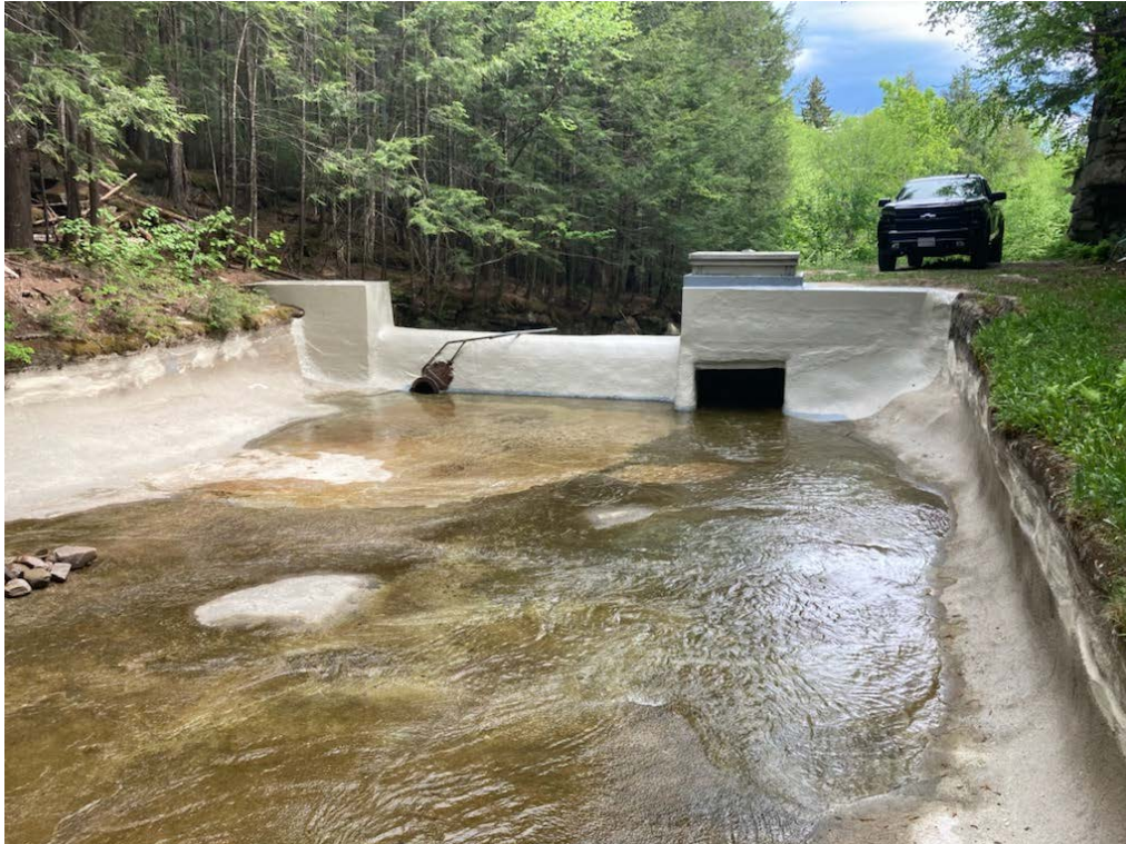
Applied Epoxy Coating to Perkins Brook Dam
