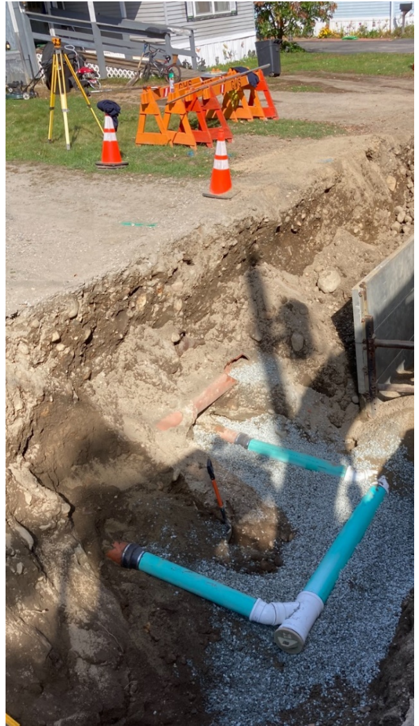
Sewer Main and Service Line Connections on Cross Street
