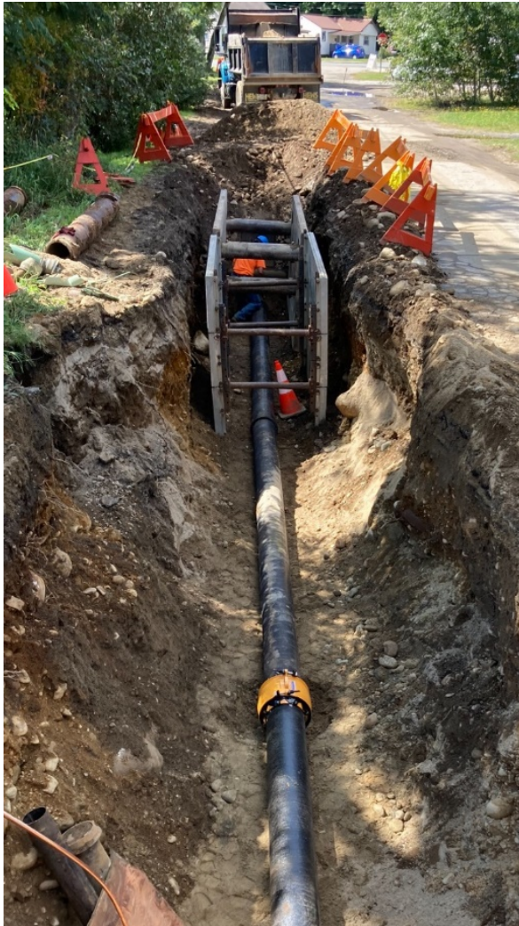
Water Main tie-in on Cross Street
