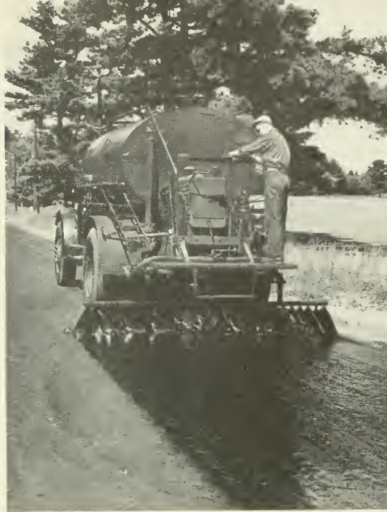
Tarring streets is a routine maintenance operation of the Highway Department
