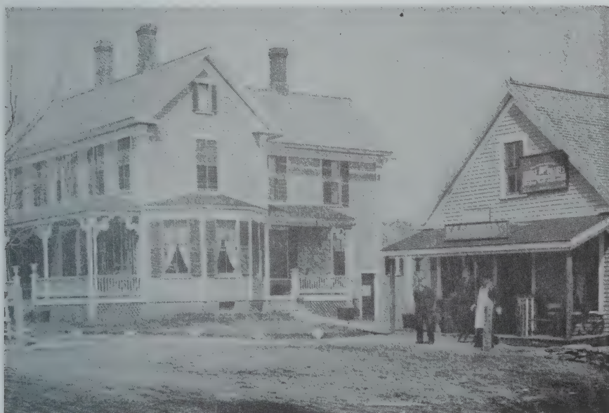
Residence & Post Office of A.F. Abbott, Moultonville, NH
