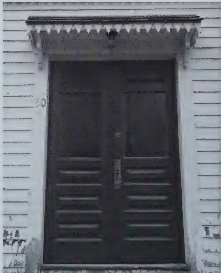
Restored doors at the East Grafton Union Church.
