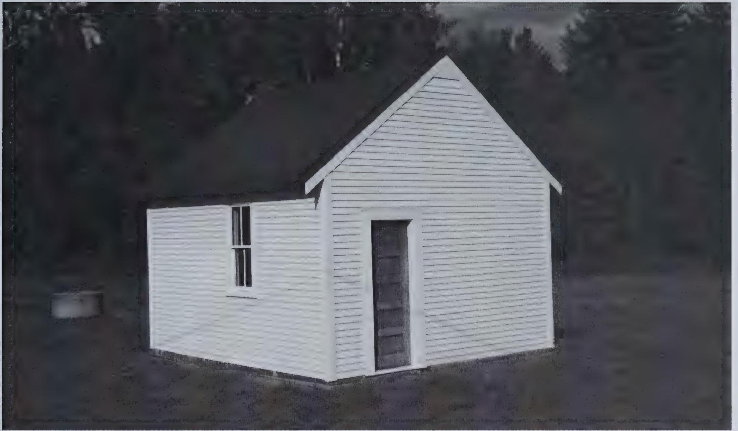
The exterior of the tramp house, newly sided and painted.
