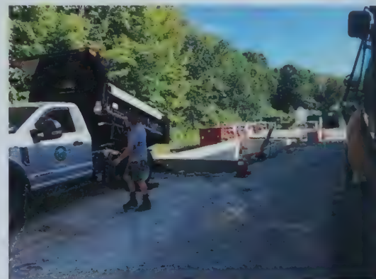
DPW site work for scale at Transfer Station
