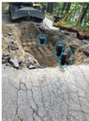
New Gate Boxes
