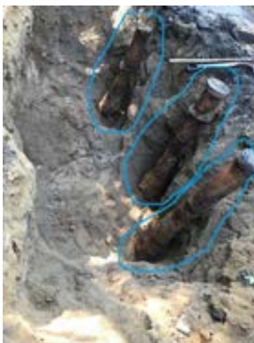
Old Gate Boxes
