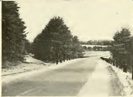
View of the new Eliot road
