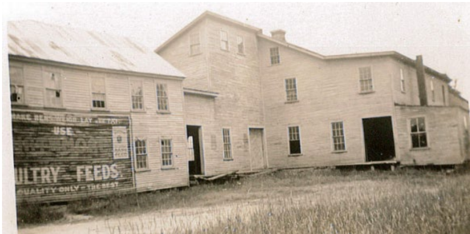
Photo of Haley's Grain Mill circa late 1920's. Haley's Grain Mill was located just north of the Rte.9/125 intersection in the current Rte. 125 right of way across from where George Calef Fine Foods is today. The State of NH purchased this property around 1936-37 and tore it down to make way for Rte. 125. Credit Barrington Historical Society Collection.
