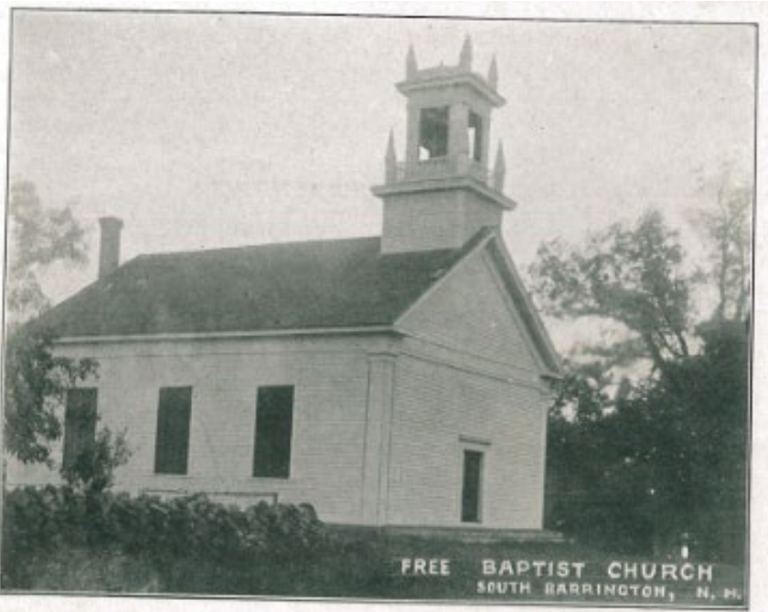
Post card of The Free Baptist Church on Beauty Hill Rd near Young Rd. Likely sold at Calef's store, building is privately owned by the Lenzi Family. Courtesy Rowell-Calef Family collection.
