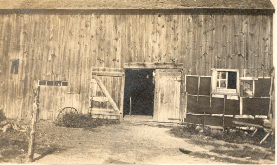
The Morley Barn on Greenhill Rd Credit: Huppe Family Collection.
