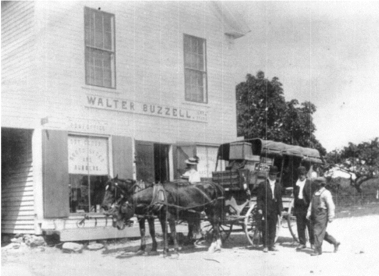
Photo of Walter Buzzell's store which was located near the intersection of Rte. 9 & Rte. 126. The sign on the front of the store is the same frame that was used for the Fire Station and is currently on display at the Public Safety Building. Circa 1920's. Courtesy Barrington Historical Society Collection.
