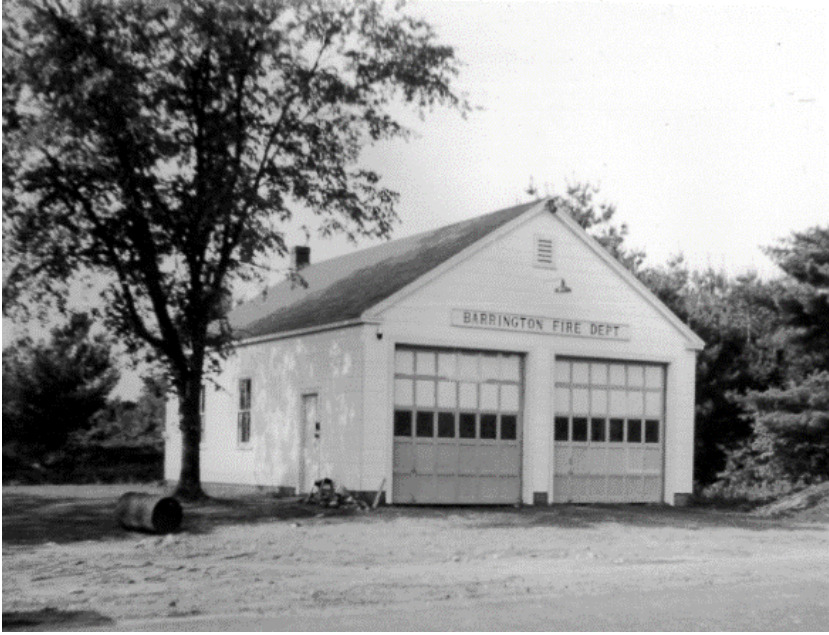
Photo of the Barrington Fire Department around the time of its completion summer circa 1947. Courtesy Barrington Firemen's Association collection.
