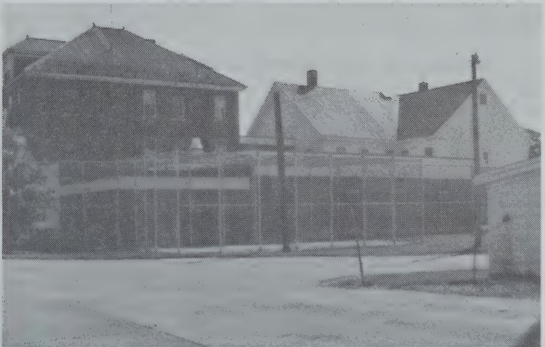
The exercise yard at the rear of the Jail and House of Corrections.
