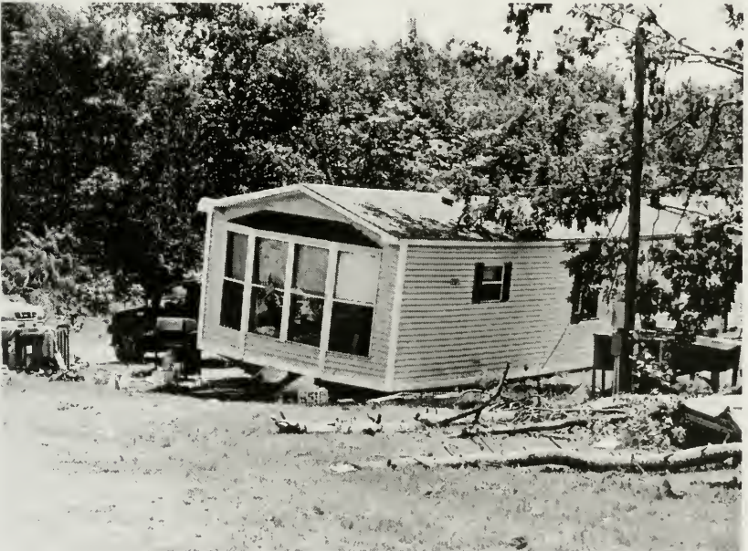
Fifield home on Shackford Corner Road, July 24, 2008. Photo courtesy of The Baysider.
