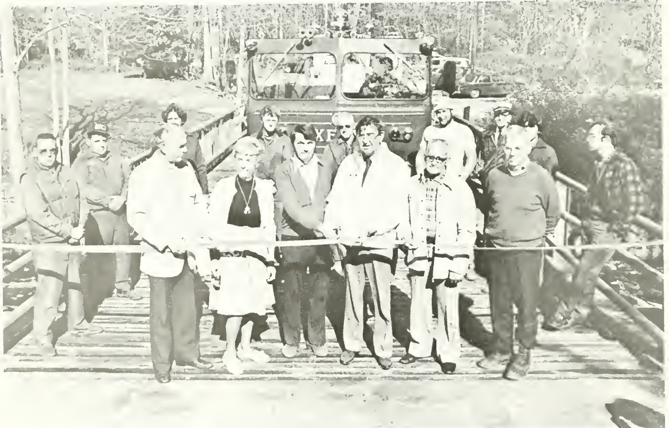
Exeter officials gathered October 21 to reopen Pickpocket Bridge, completely rebuilt by the highway department during late summer.
