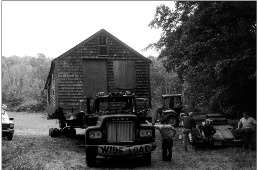
THE BUILDING AWAITS ITS MOVE ON A FLATBED
