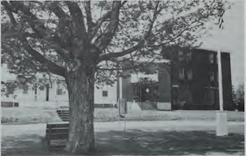
A view of the Carroll County Jail & House of Correction.
