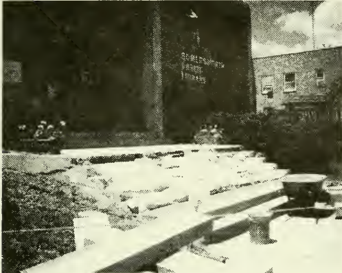
Library steps under renovation
