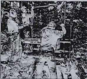
Cable Car Installation
