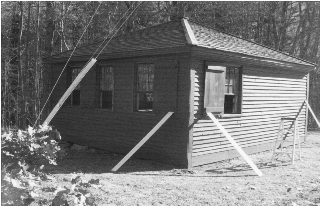
North-west corner after done painting
