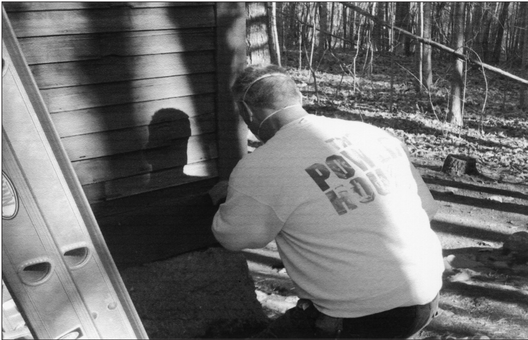
Volunteer, Mark Raumikaitis, scraping paint from south-eastern corner
