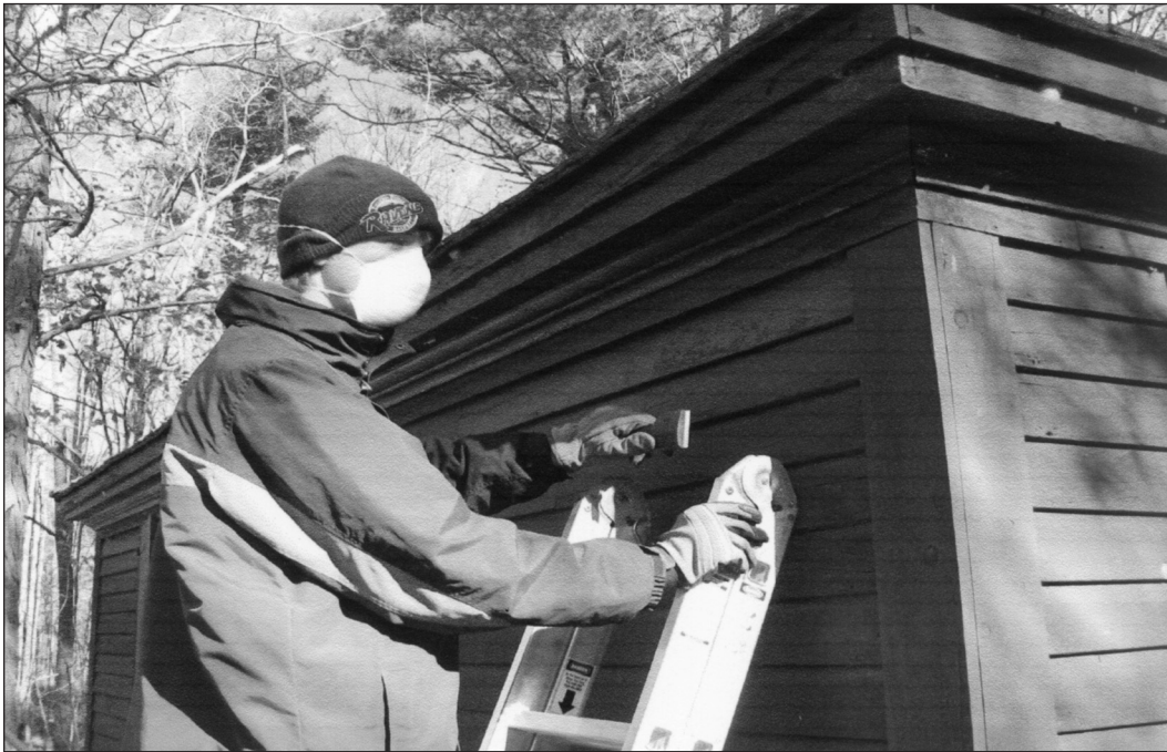
Volunteer, Drew Mather, scraping paint from front of building
