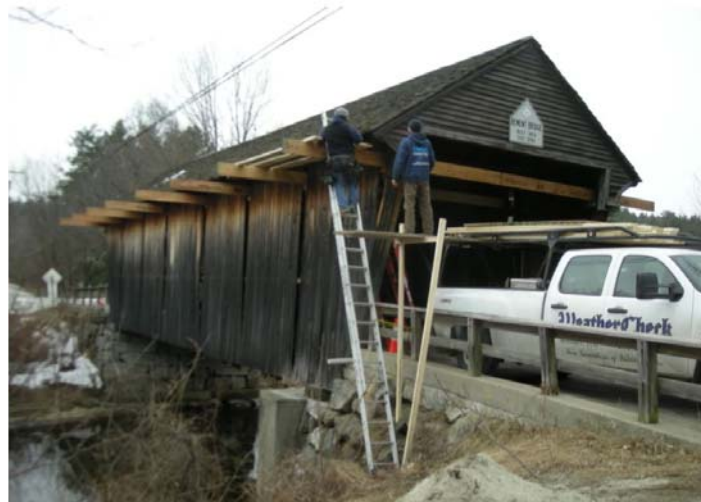
Preparation to install new roof on Bement Bridge
