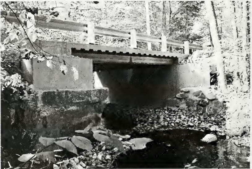
Pineo Road Bridge repaired after the flood of 2006.
