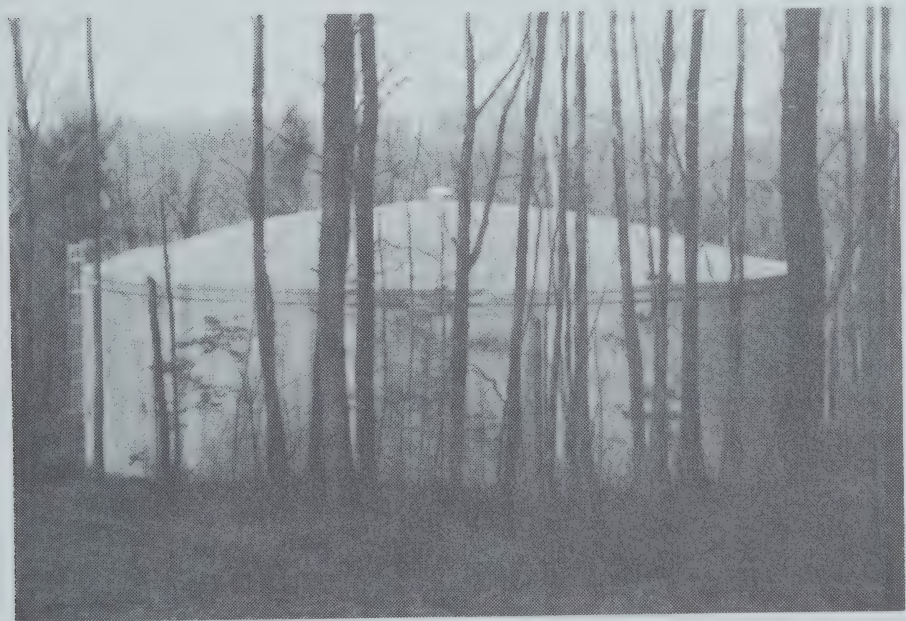
Water Storage Tank
